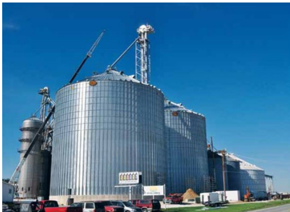
◀ Watch Communications Vertical Asset
